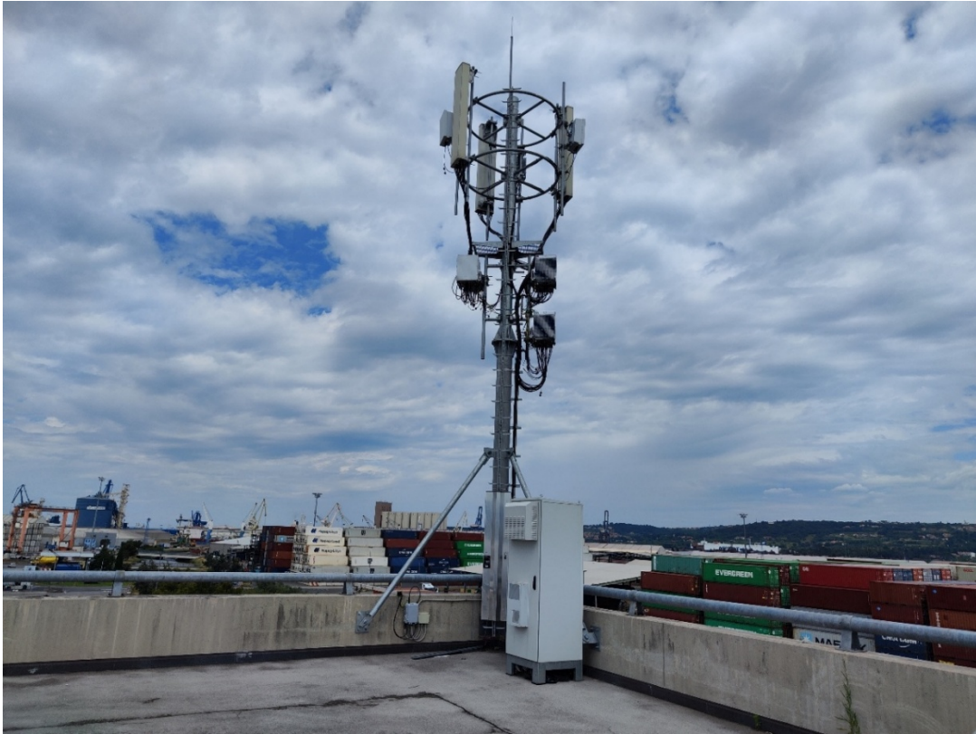
Figure 12. Locations of base station at the corner of the parking garage.
